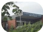
Parking to be limited at Congleton War Memorial Hospital from 2nd to 13th December as work continues on new Community Diagnostic Centre :: East Cheshire NHS Trust
